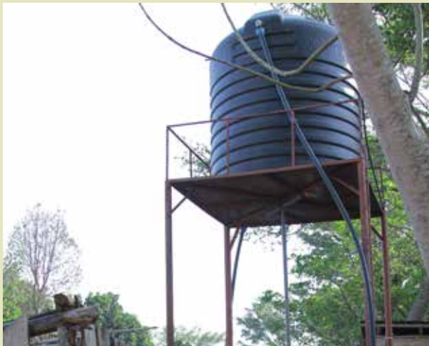
Overhead water reservoir
